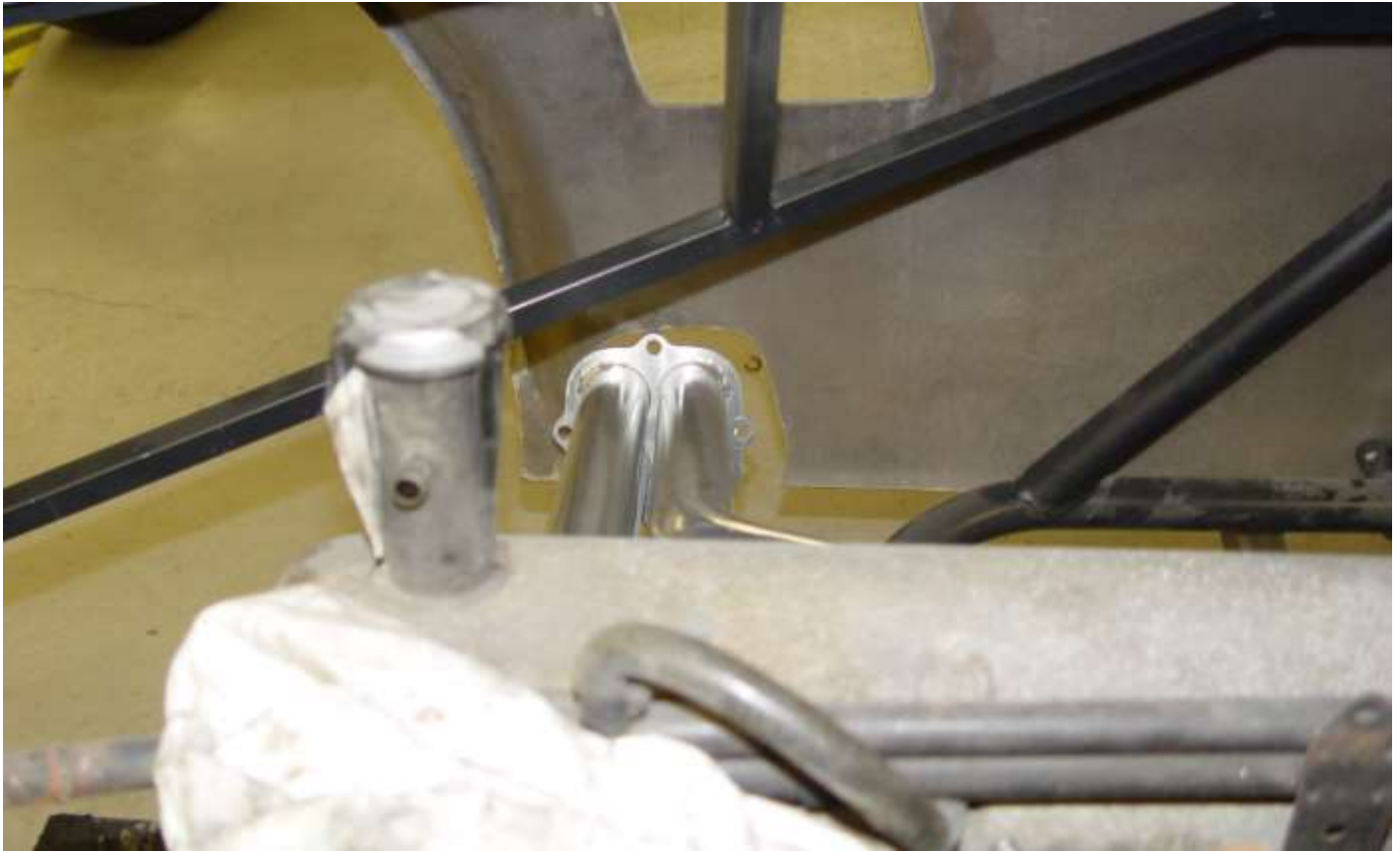
PASSENGER SIDE, VIEW FROM TOP, INSIDE ENGINE COMPARTMENT
